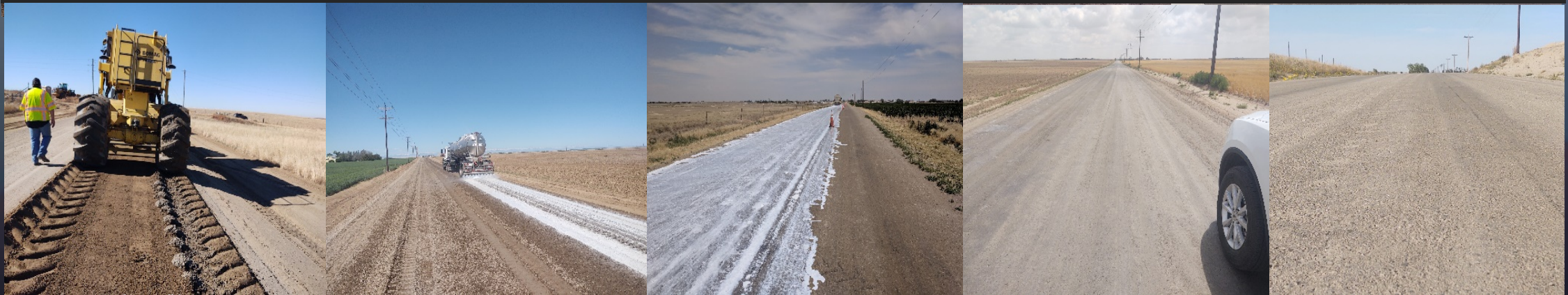
Saturate Coat/Grade/Compact
