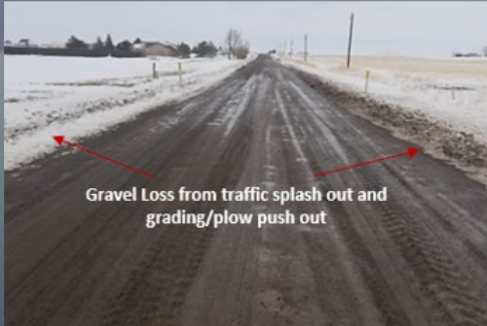
Saturated road = gravel loss and short lifecycles
