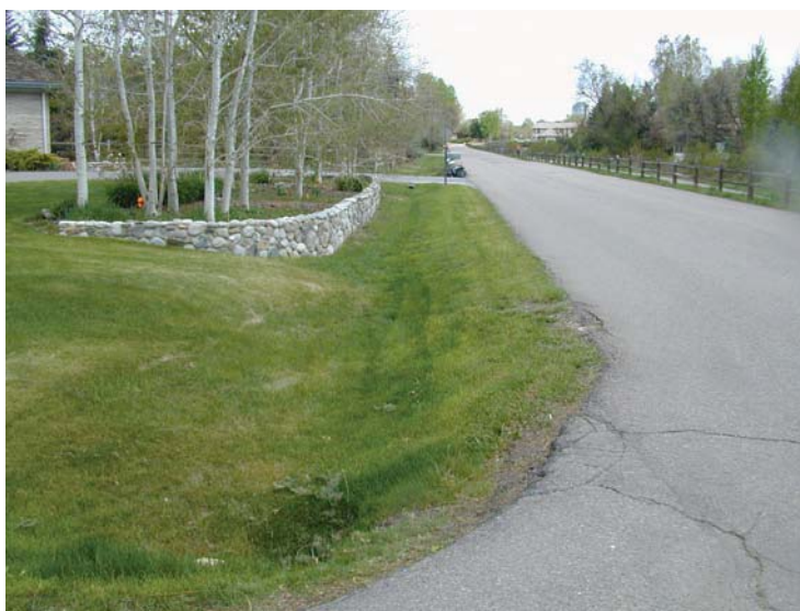
Photograph GS-1. This grass swale provides treatment of roadway runoff in a residential area. Photo courtesy of Bill Ruzzo.
