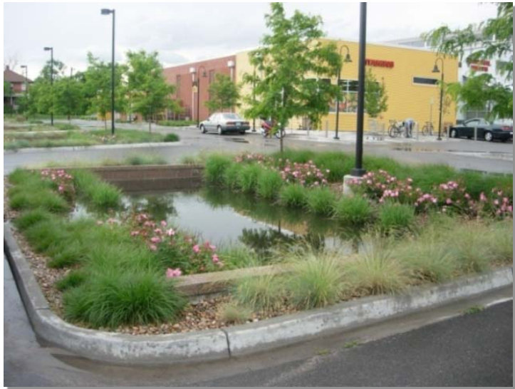
Photograph EDB-4. A series of landscape islands connected by culverts provide water quality and flood control for this site.
