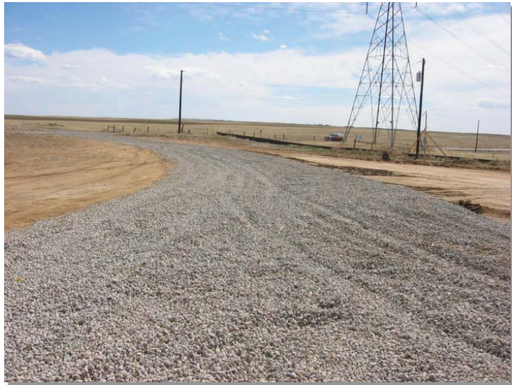
Photograph SCR-1. Stabilized construction roadway.
