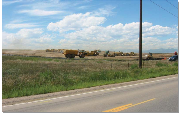
Photograph VB-1. A vegetated buffer is maintained between the area of active construction and the drainage swale. Photo courtesy of WWE.
