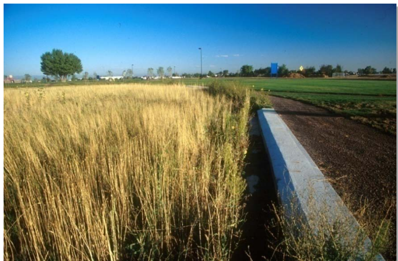
Photograph GB-2. This level spreader carries concentrated flows into a slotted pipe encased in concrete to distribute flows evenly to the grass buffer shown left in the photo. Photo courtesy of Bill Wenk.
