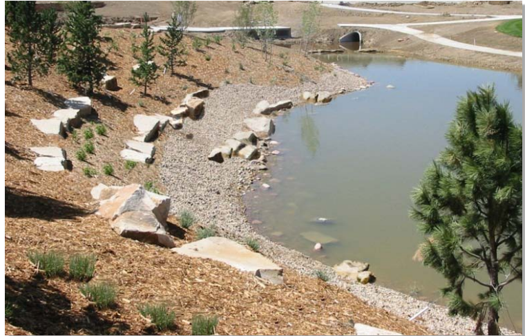
Photograph RP-4. (altered photo) Variations in slope and texture around the pond are brought together by mass groupings of local stone boulders. The boulders are placed intermittently around the pond in groups and interspersed with plantings. Photo courtesy of Design Concepts. Note: A minimum 4-foot vegetated buffer (littoral zone) is recommended to strain surface flow into the pond, protect the banks by stabilizing the soil at the edge of the pond, and provide biological uptake.
