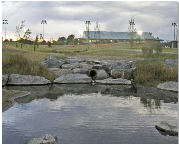
Photograph RP-3. (altered photo) When incorporating rock into a structure, use other matching, functional rock to prevent the structure from looking out of context. Photo courtesy of Design Concepts.
