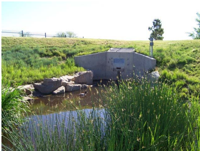
Photograph EDB-2. The initial surcharge volume of this EDB is contained within the boulders that surround the micropool.
