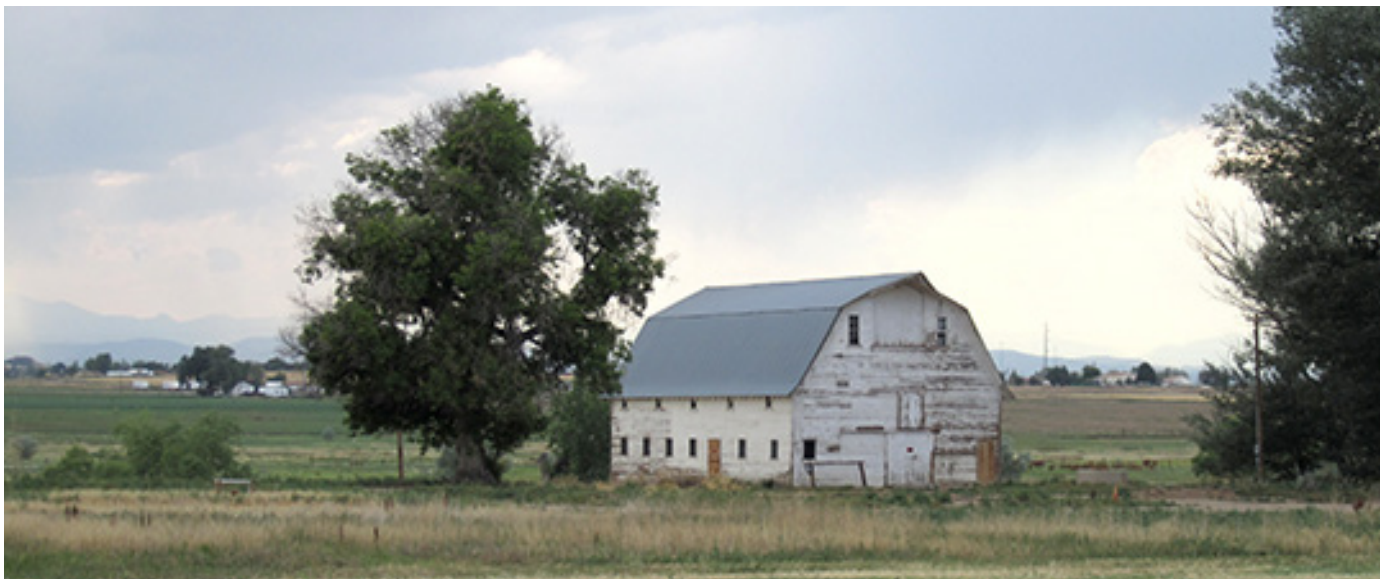
Restoration is planned for a historic barn located within protected open space.
