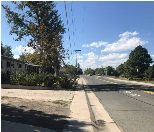
Undersized sidewalk on 60th Avenue.
