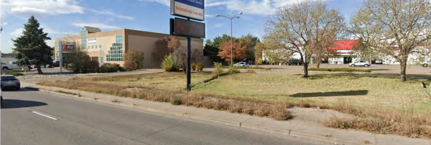
Figure 7: Example of Narrow Sidewalk on Federal Boulevard
